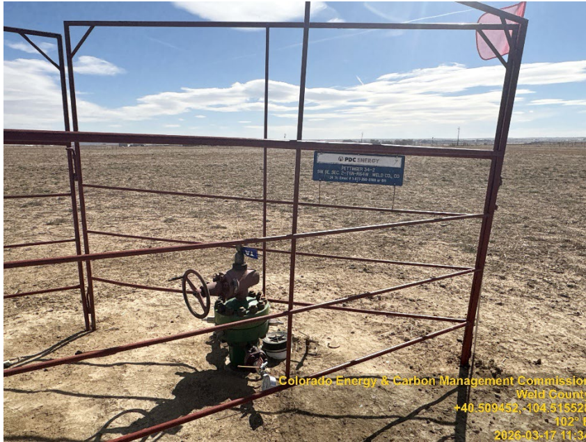
Photo #1 Pettinger 34-2 (123-23591) Wellsite Temporarily Abandoned | TA
