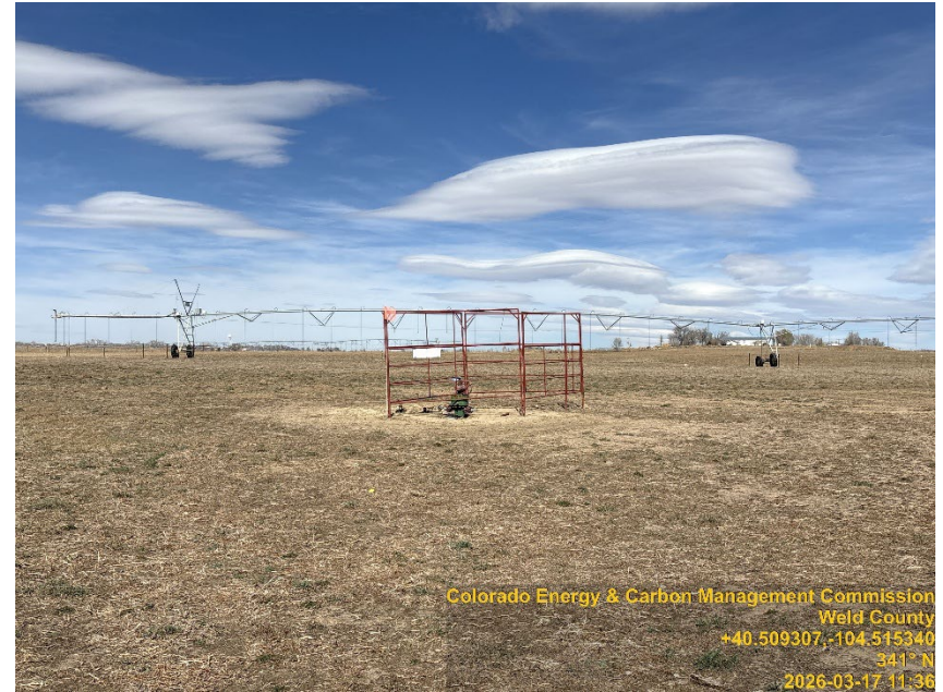
Photo #2 Pettinger 34-2 Wellsite Temporarily Abandoned | TA macro view
