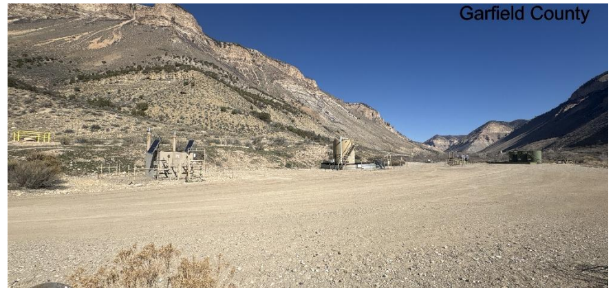
South East corner of location.
