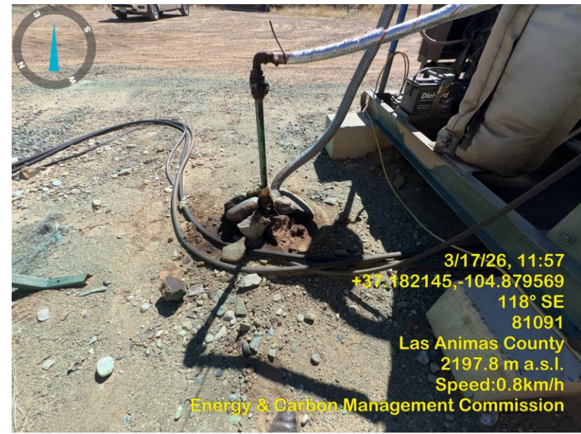
Photo 12 Stained soil by skid engine gas valve.
