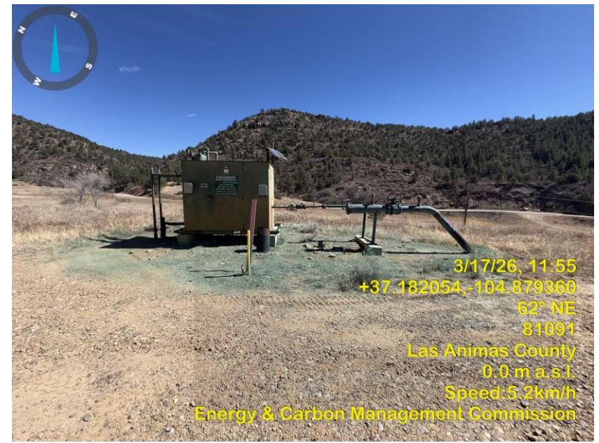
Photo 4 Gas Meters & Pig station.
