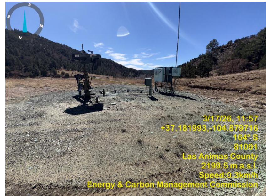
Photo 14 Wellhead & Automation control panel.
