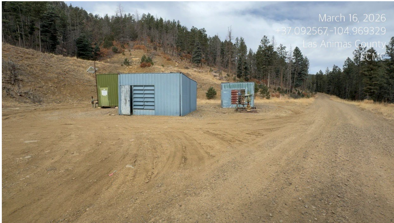
Photo 2. Facing northwest at the location.
