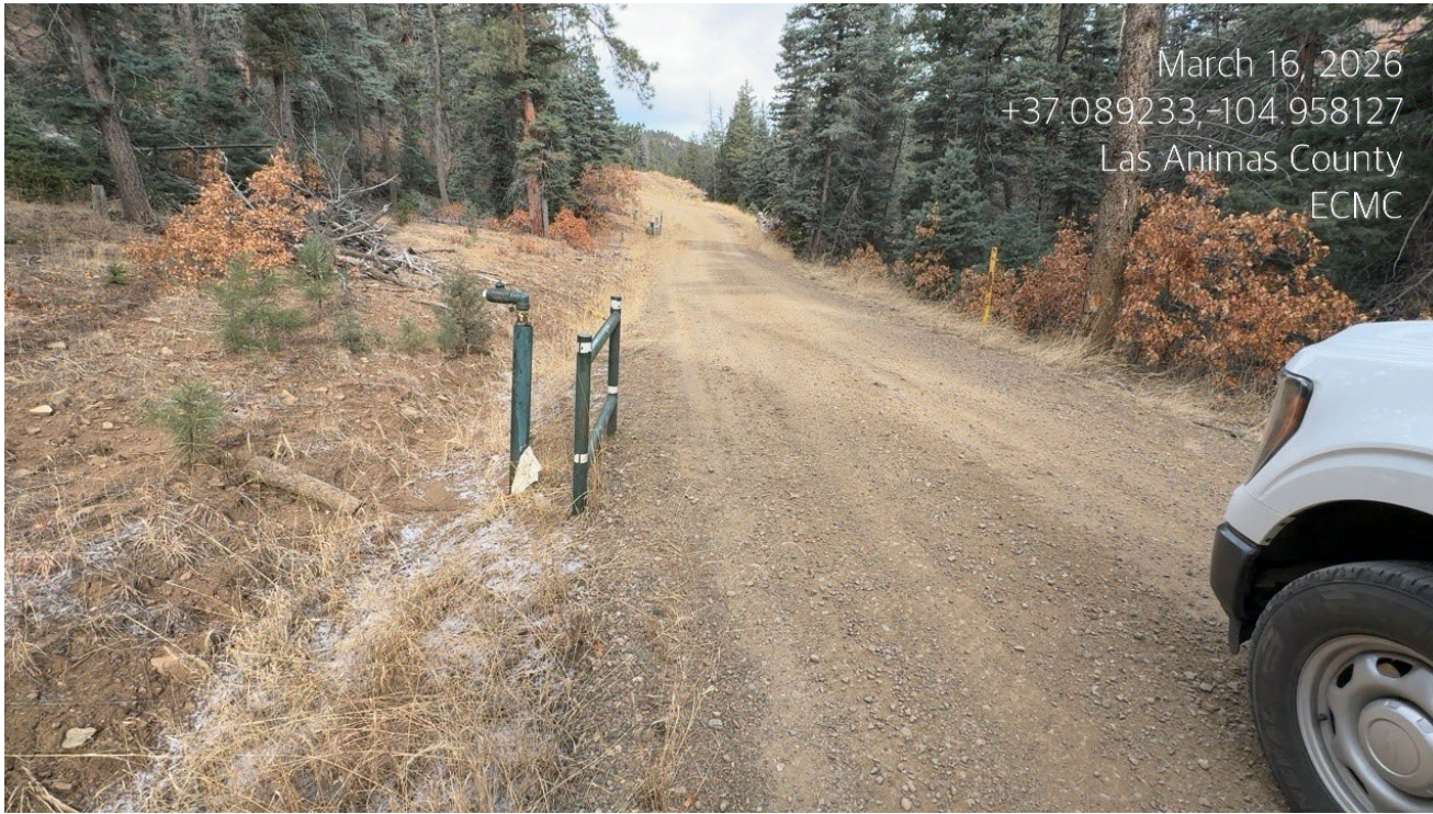
Photo 1. Facing northwest along the access road.
