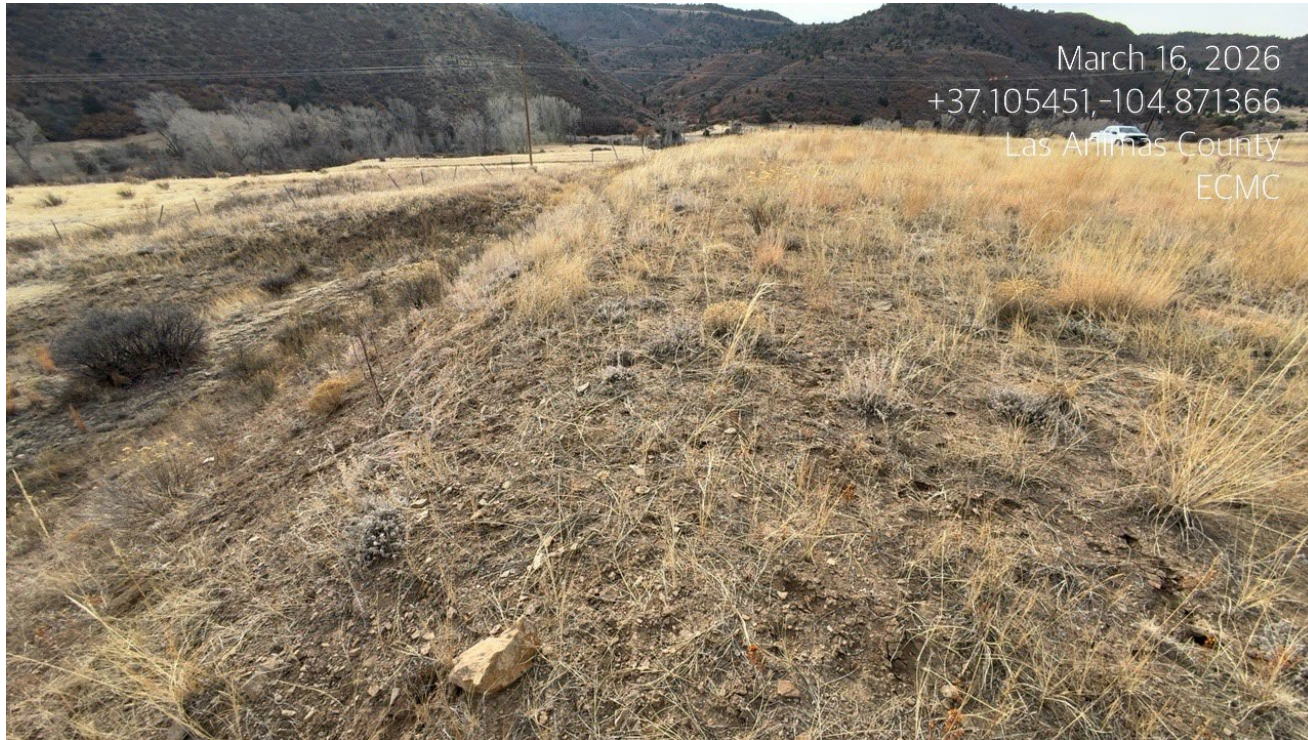
Photo 4. Facing southeast along the fill slope.
