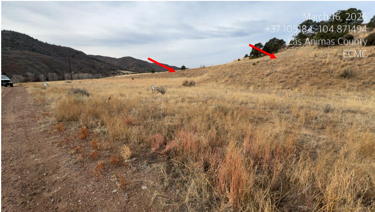
Photo 3. Facing southwest at the location. The location has not been contoured back to original contours shown at red arrows. .
