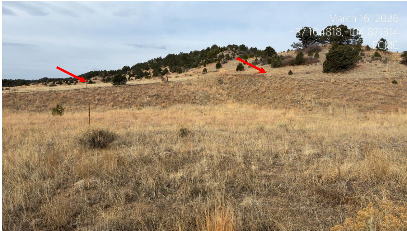
Photo 2. Facing west at the location. The location has not been contoured back to original contours shown at red arrows.
