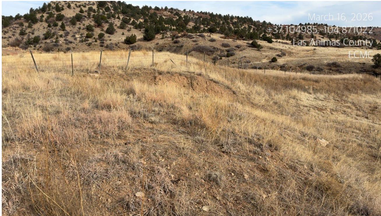
Photo 5. Facing north along the fill slope
