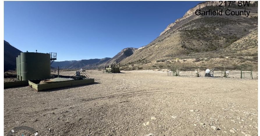
North East corner of location.
