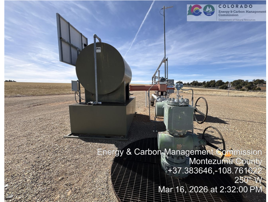
6. Wellhead, stainless flowline, 1000 gallon produced water/diethylene glycol tank atop secondary containment tank with expanded metal screen, and solar telemetry.
