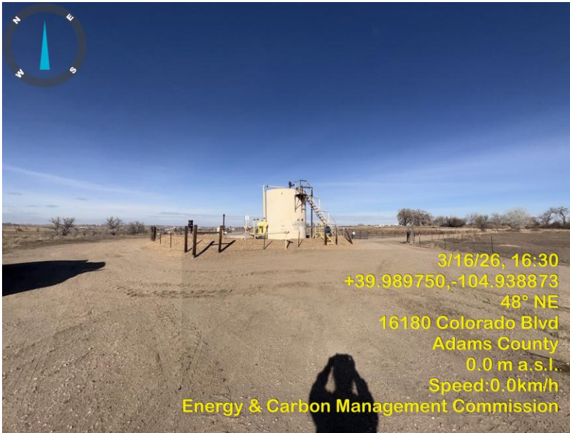
Photo 5 Tank battery location.
