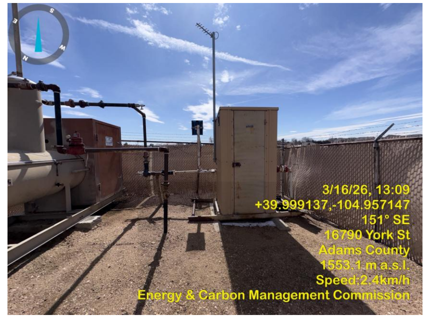
Photo 10 Gas Meter Run.
