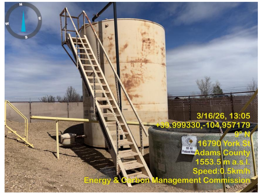
Photo 6 Tank battery.
