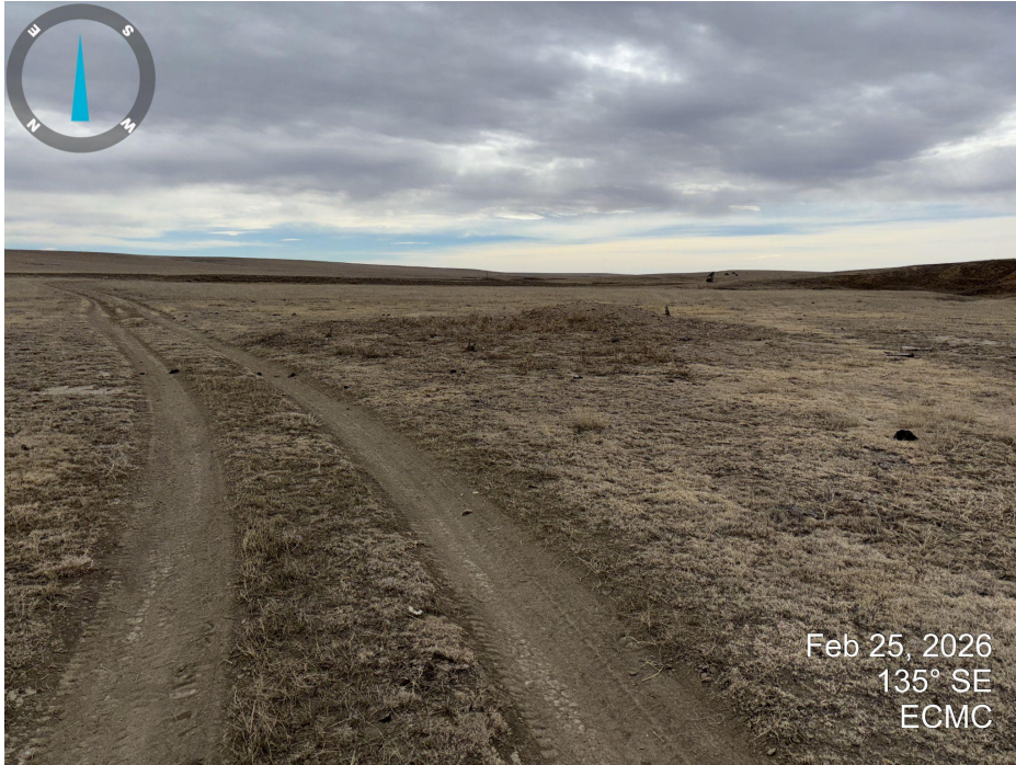
Photo 1. Looking southeast across the well location. An approximately 3ft pile of gravel/soil is present over the wellbore. No oil and gas equipment is present on the surface.
