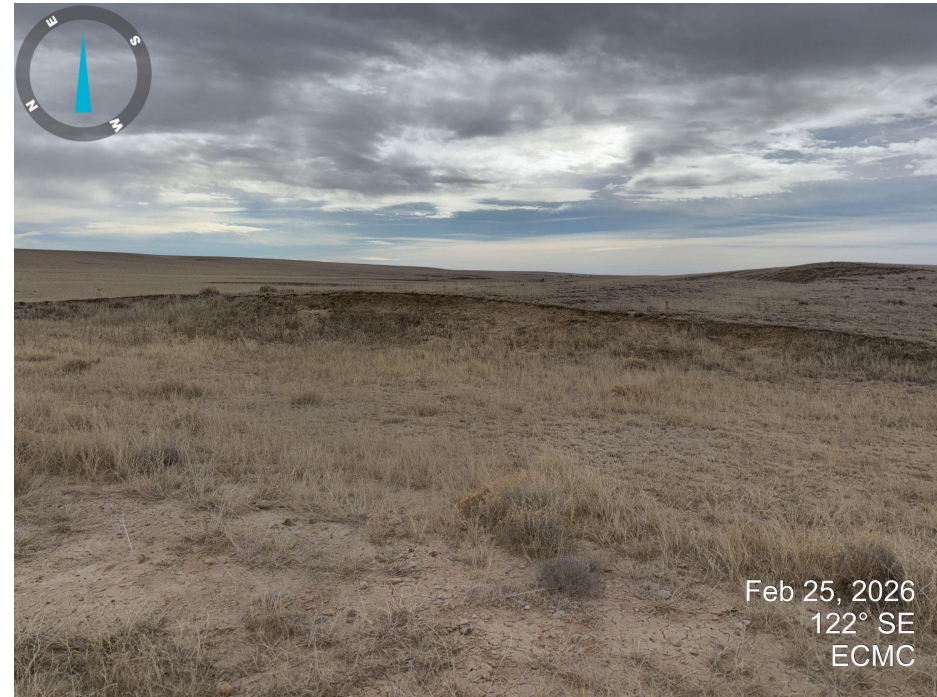
Photo 6. Looking east across the tank battery location. The tank battery has not been recountured to match the surround terrain. The east cut slope does not appear to be stabilized and does not have vegetation establishment that is reflective of the surrounding area.
