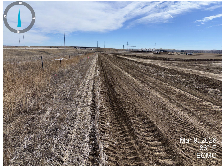
Photo 10. Looking east down the north side of the location. A ditch and berm is present on a portion of this side of the location. Th ditch and berm transitions to filtrex waddles near the east side.
