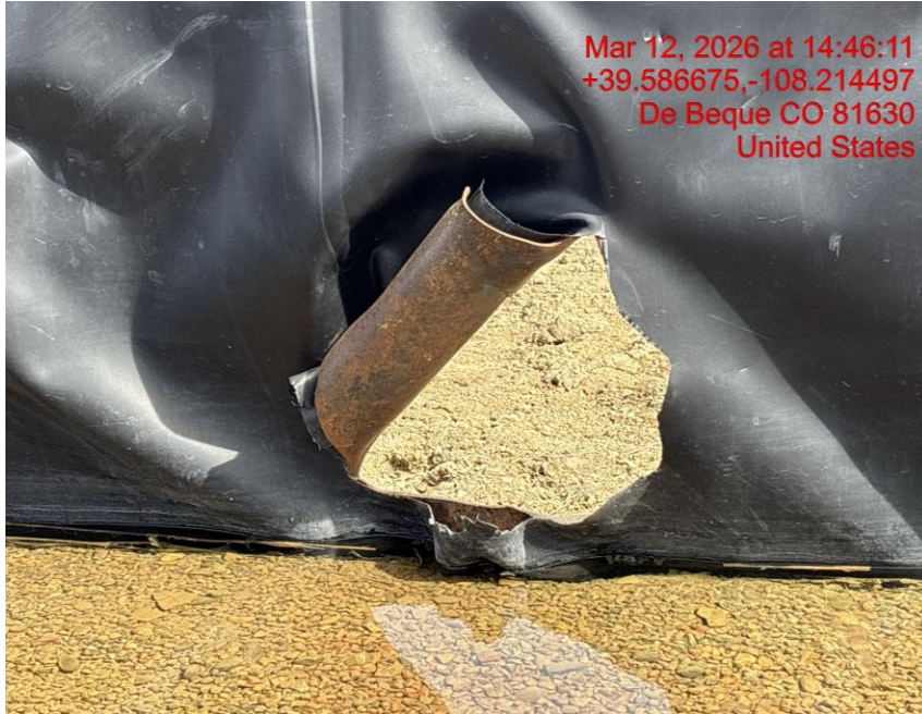
Punctured Berm Wall – Photo #03059
