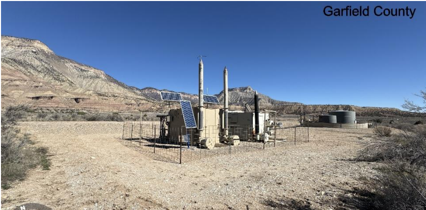
South West corner of location.
