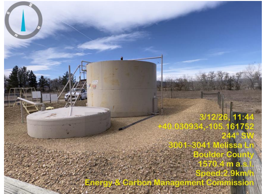
Photo 6 Tank battery.
