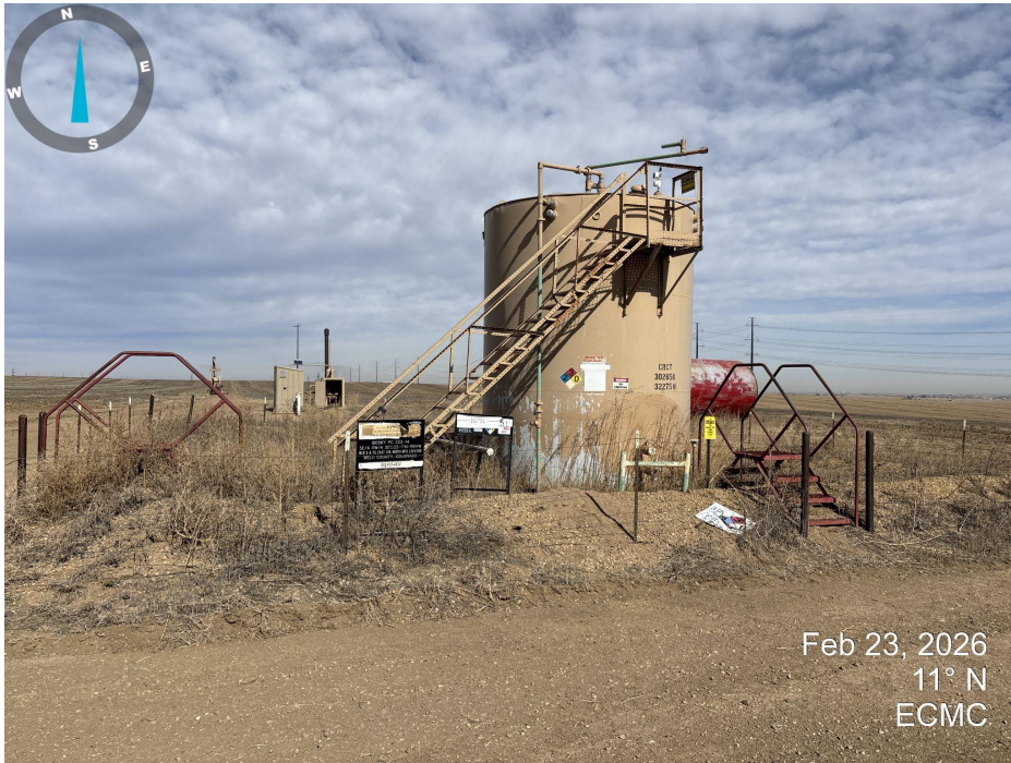
Photo 1. Photo taken looking north across tank battery. Undesirable weedy annual plant species are present throughout location. (Kochia, Russian thistle).
