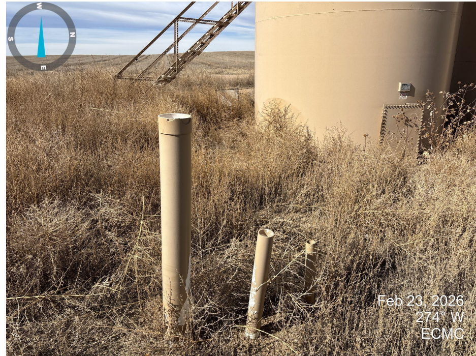
Photo 8. Uncapped pipes without wildlife exclusion devices at tank battery.
