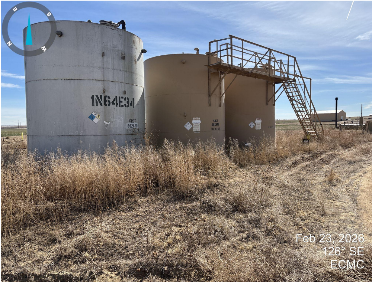
Photo 9. Looking south across tank battery. Undesirable weeds are overgrown on location.
