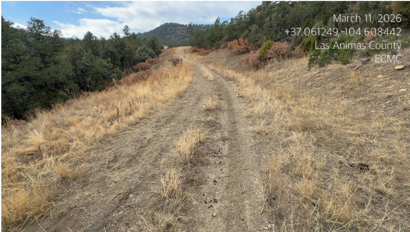
Photo 2. Facing southwest along the access road. The access road is stabilized and maintained in good condition.
