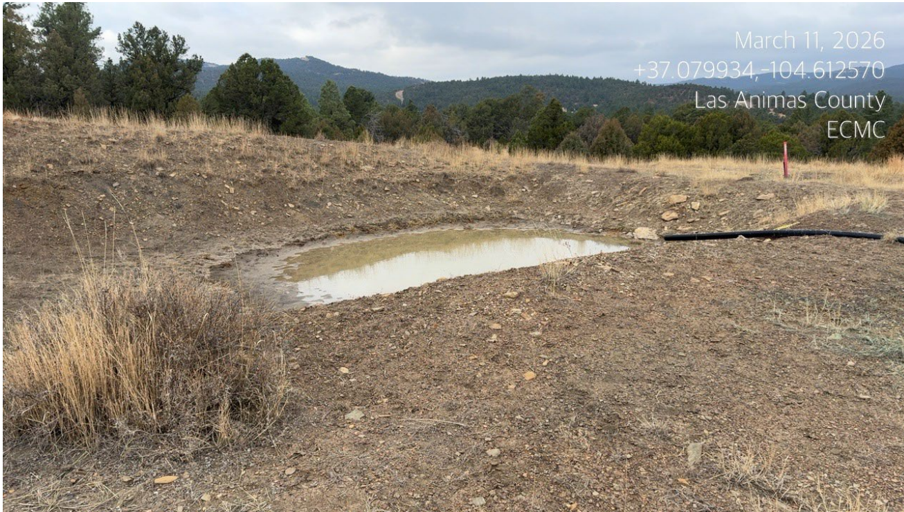
Photo 5. Facing toward PW pit.
