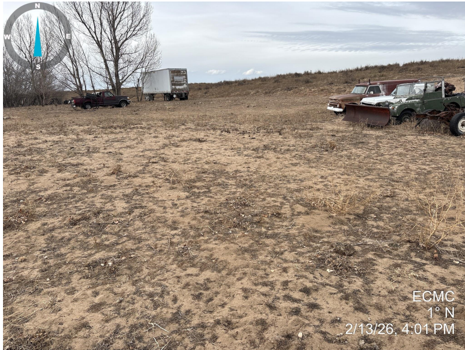
Photo 1. Photo taken of the multi-well location, facing north. Photo illustrates that final reclamation activities appear to have taken place, but vegetation establishment does not meet Rule 1004 standards.
