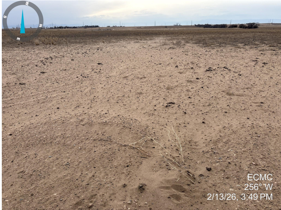
Photo 6. Photo taken of the access road to the well location, facing west. Photo illustrates that the access road to the location does not meet Rule 1004 standards as gravel and bare ground were observed.
