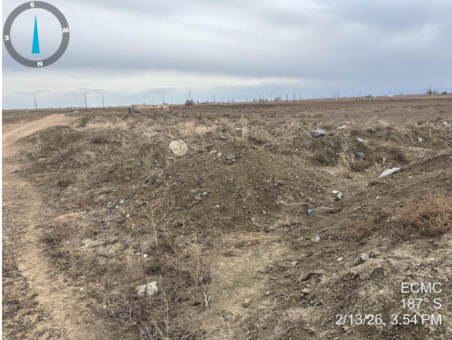
Photo 7. Photo taken of the tank battery location, facing south. Photo illustrates that final reclamation does not meet Rule 1004 standards at the tank battery location and the location is in use by the landowner.
