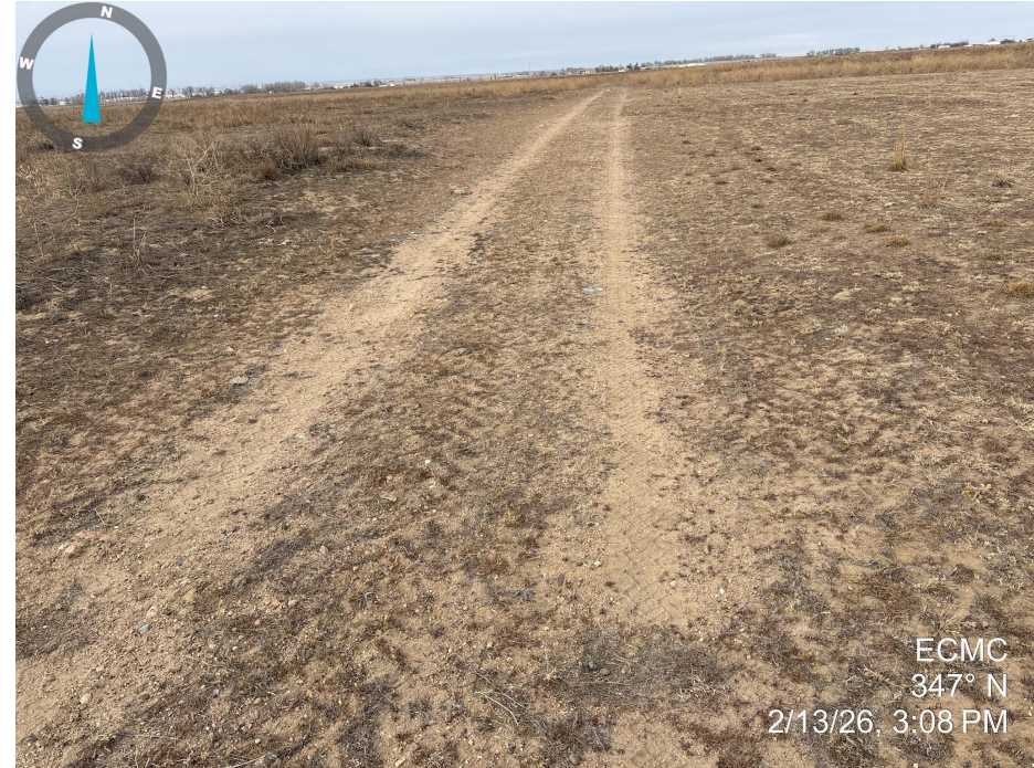
Photo 10. Photo taken of the access road to the tank battery location, facing north. Photo illustrates that final reclamation activities appear to have taken place, but vegetation has not established to Rule 1004 standards and bare ground remains across the access road.
