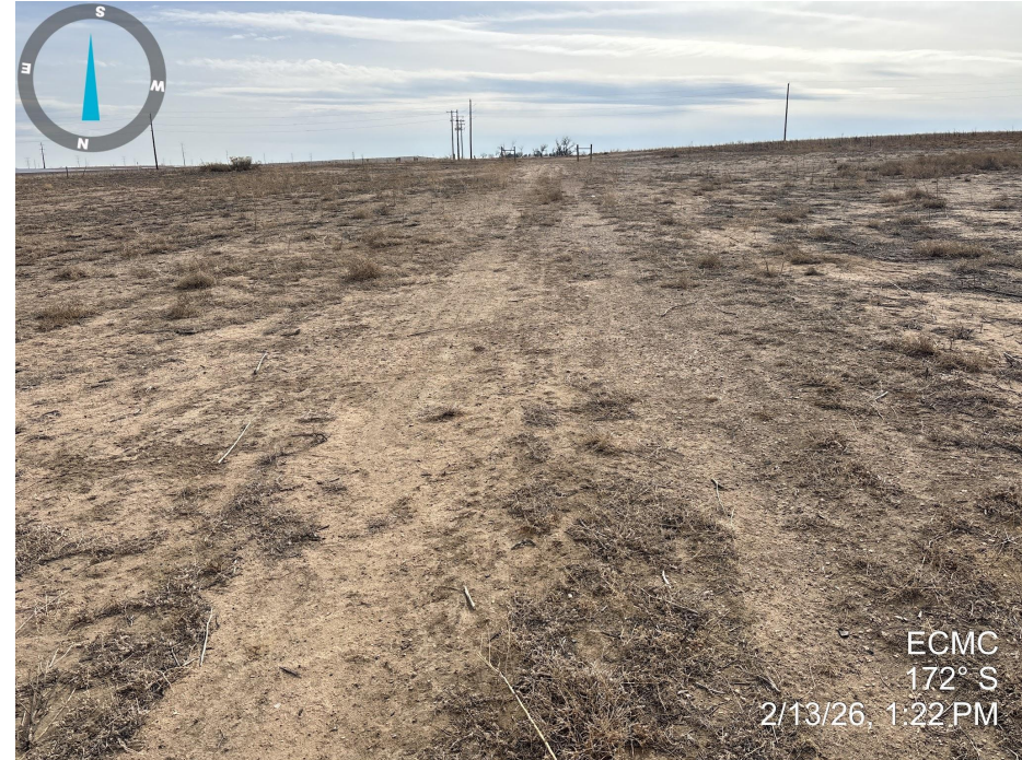
Photo 6. Photo taken of the access road to the location, facing south. Photo illustrates that vegetation has not established to Rule 1004 standards.
