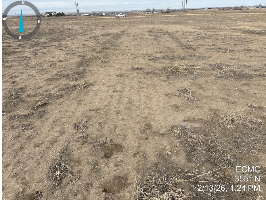
Photo 9. Photo taken of the tank battery location, facing north. See comments under Photo 7.
