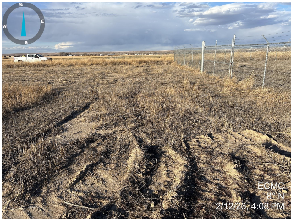
Photo 6. Photo taken of the tank battery location, facing north. Photo illustrates that final reclamation activities do not appear to have taken place at the location as gravel, bare ground, and weedy annual vegetation were observed across the location.
