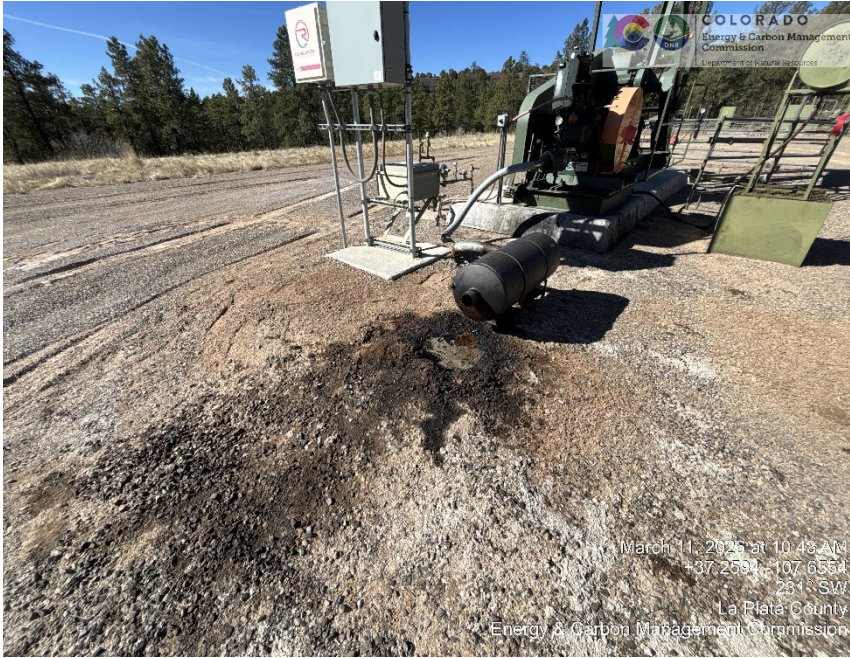
EXHAUST LEAKING ONTO LOCATION
