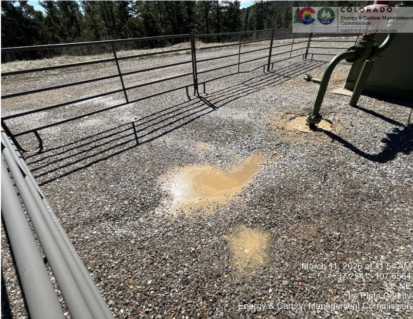
FLOW LINE LEAK
