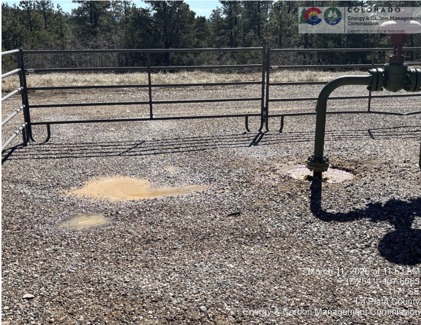
FLOW LINE LEAK
