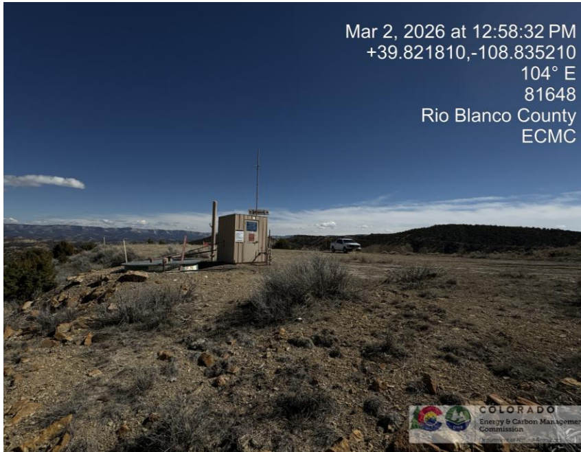
Photo # 2663 NW corner of location
