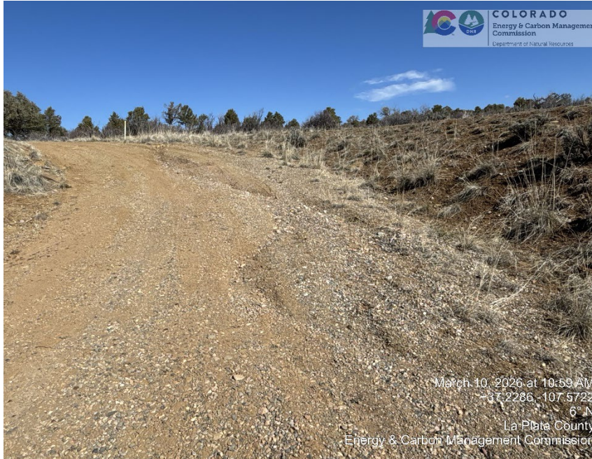
ENTERANCE OF LOCATION HAS DEEP RUTS FROM STORM WATER EROSION
