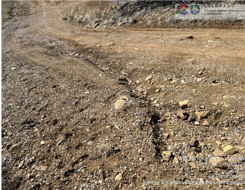
ENTRANCE OF LOCATION HAS DEEP RUTS FROM STORM WATER EROSION
