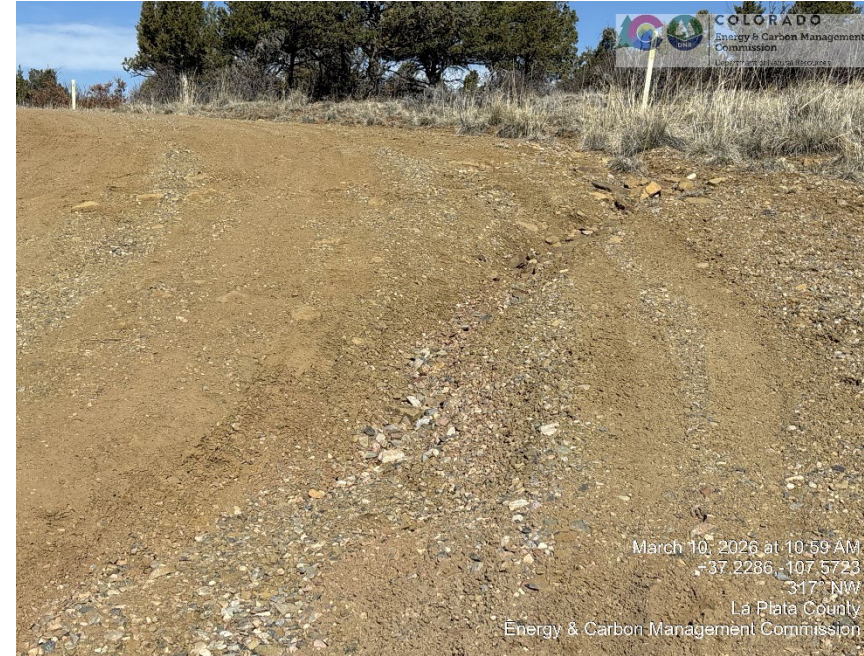
ENTERANCE OF LOCATION HAS DEEP RUTS FROM STORM WATER EROSION
