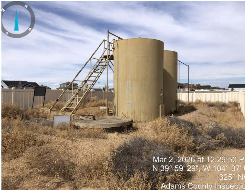
Photo #1 Tanks, vault and weeds throughout location (in and out of berms).
