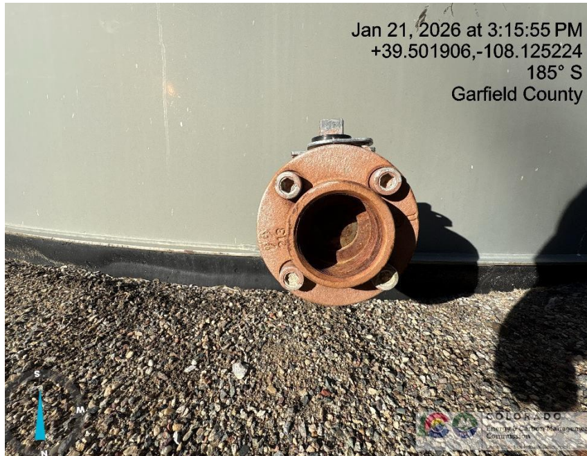
Photo # 3598 From inspection/audit 708908346 conducted on 01/21/2026 - Open ended load line
