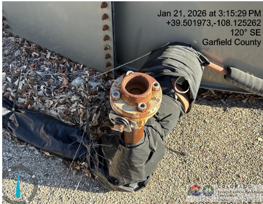
Photo # 3599 From inspection/audit 708908346 conducted on 01/21/2026 - Open ended load line
