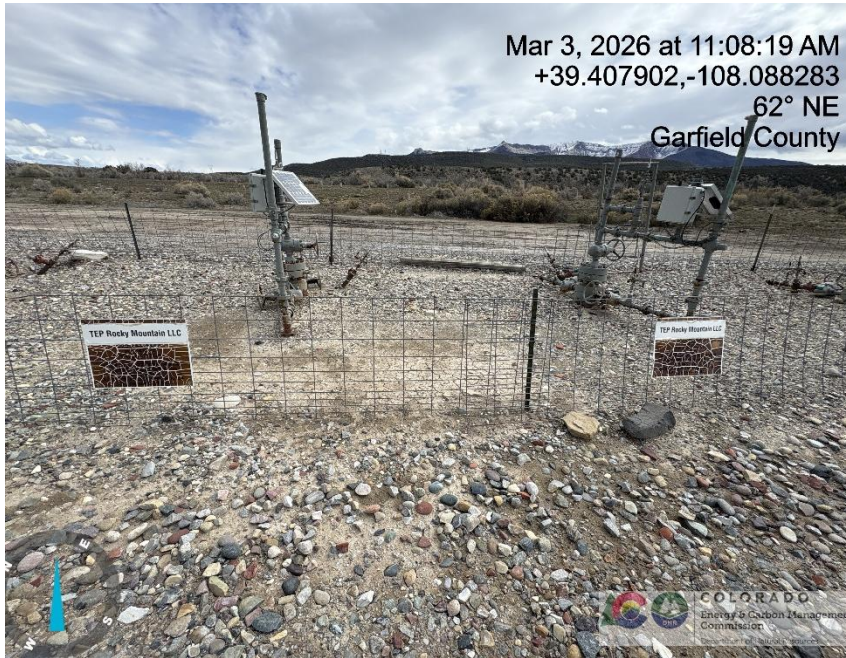
Photo # 4544 Wellhead signs damaged & illegible
