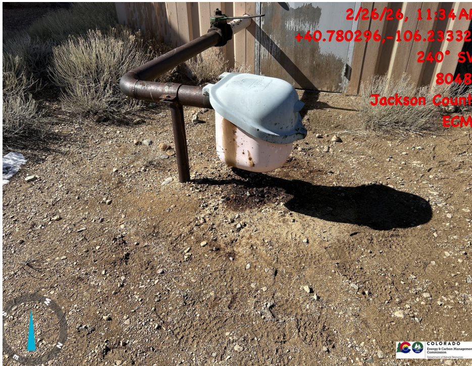
Recent inspection/audit of staining under load out bucket
