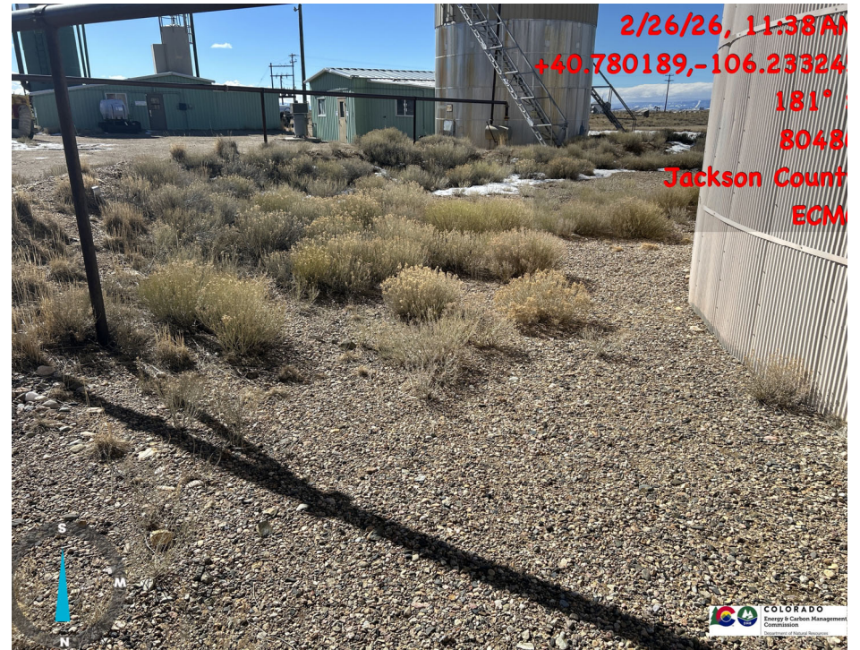
Weeds throughout secondary containment
