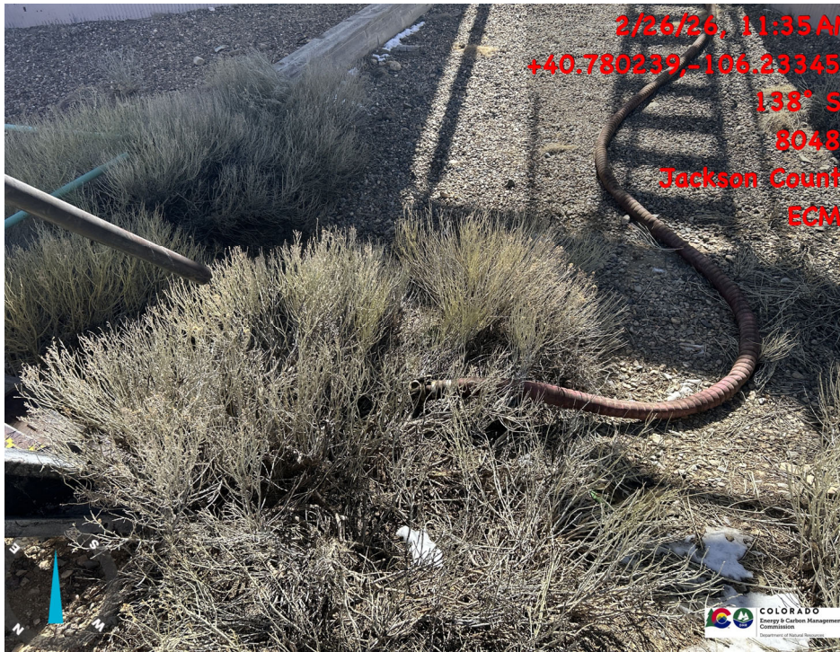
Weeds throughout secondary containment and debris
