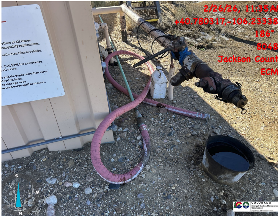
Recent inspection/audit of bucket with crude and staining
