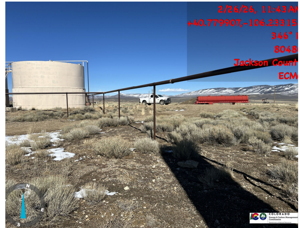
Lines from tanks that go to ECD
