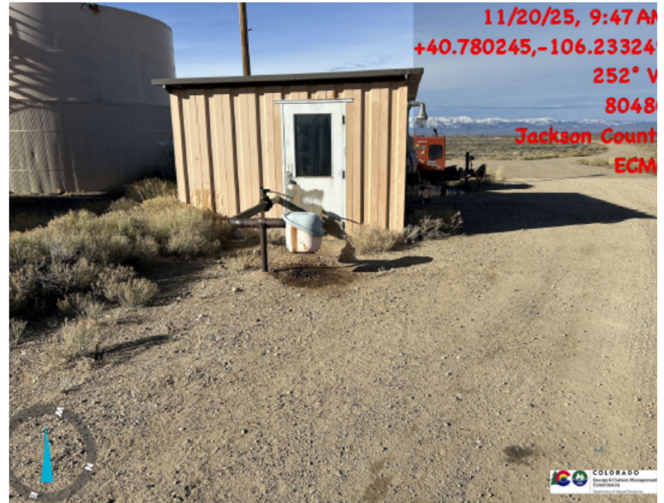
Previous inspection/audit of staining under load out bucket
