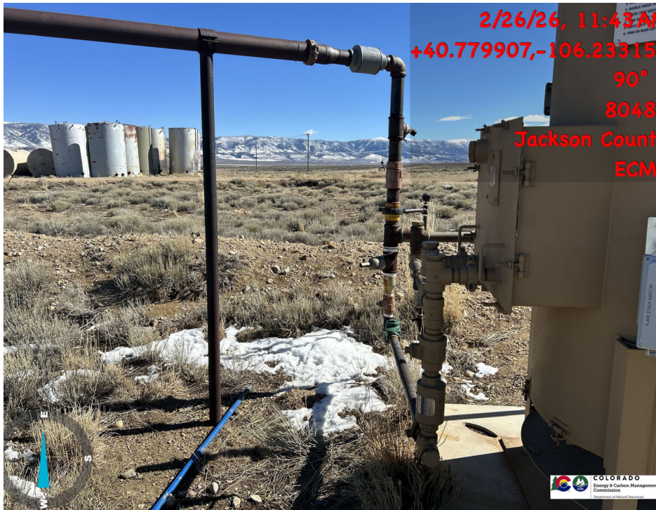
Lines from tanks that go to ECD and not metered
