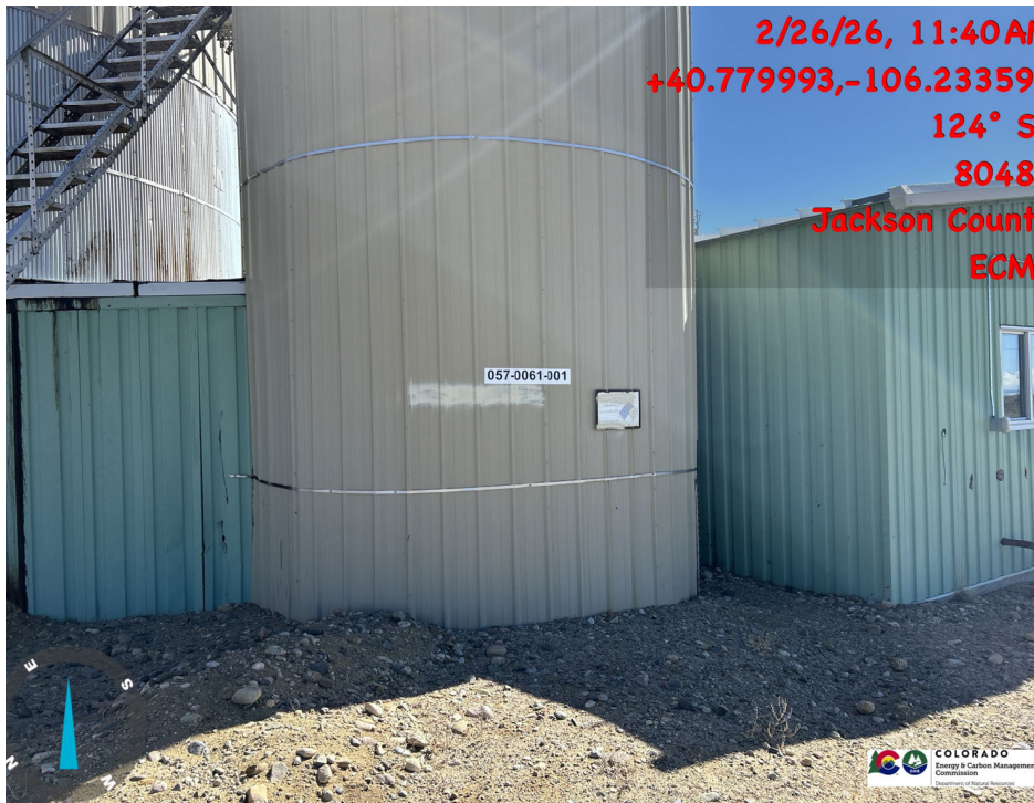
Recent inspection /audit of illegible tank labeling
