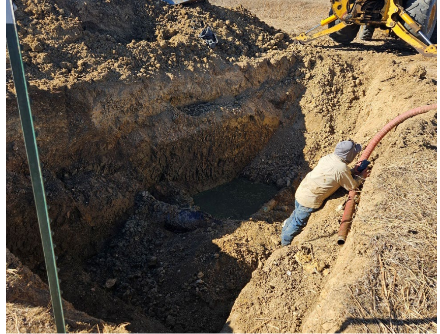
Operator personnel within excavation at spill location.
