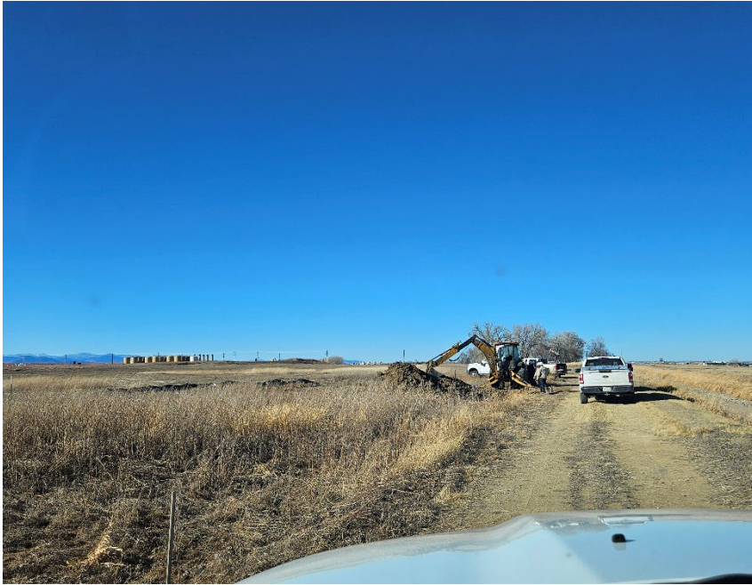
Operator personnel observed on location, in the process of excavating soil.
