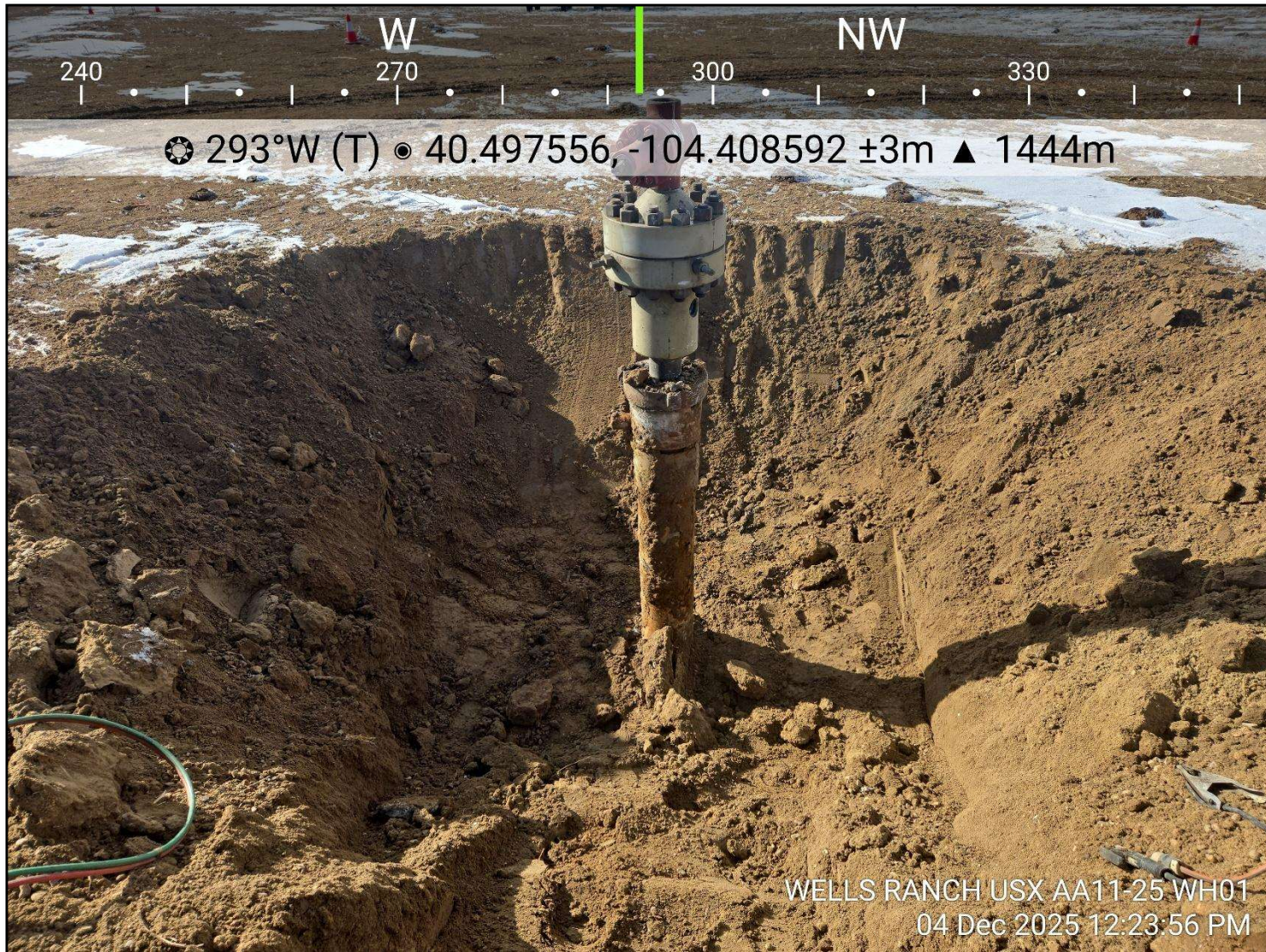
Photo 1: View of wellhead excavation extent, facing west-northwest
