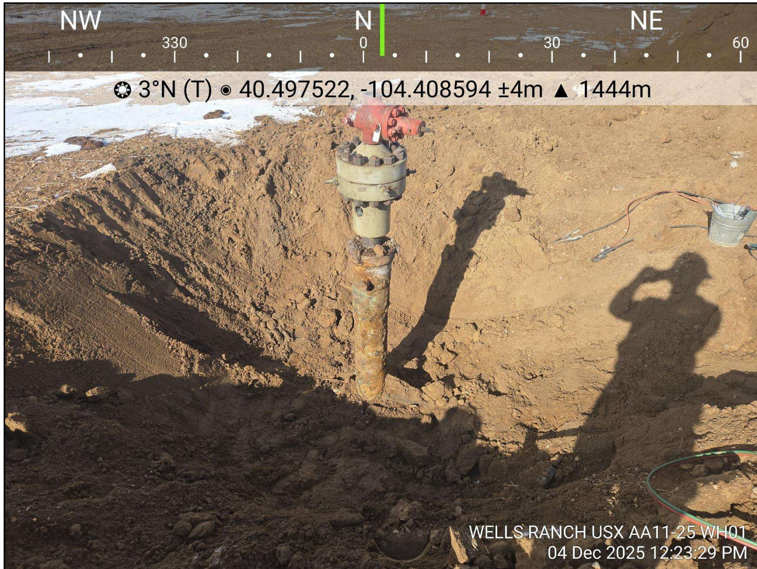
Photo 4: View of excavation extent, facing north
