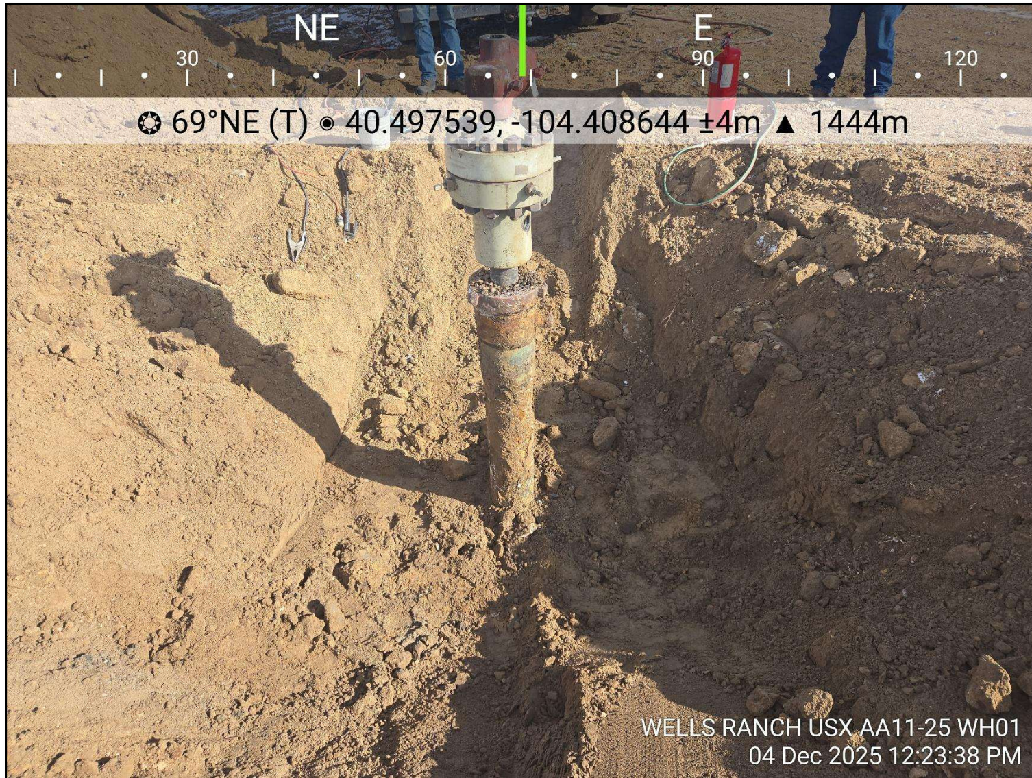
Photo 3: View of excavation extent, facing east-northeast
