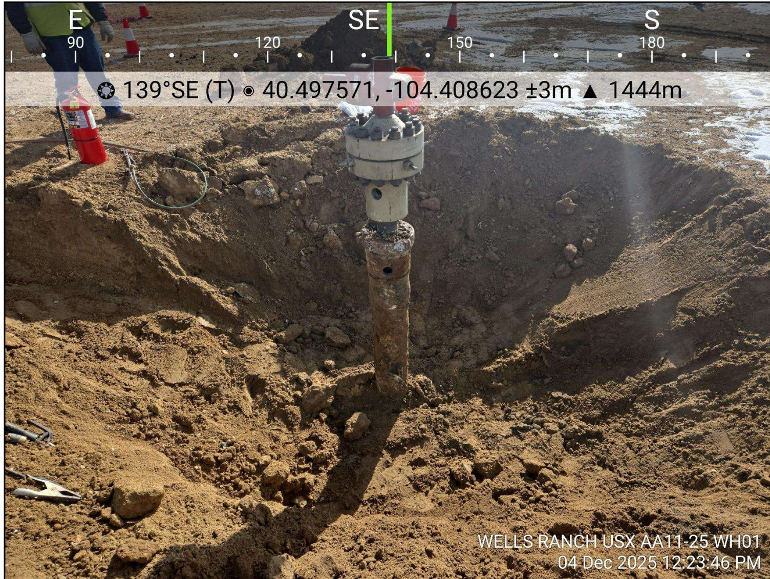
Photo 2: View of wellhead excavation extent, facing southeast
