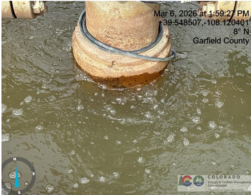
Photo # 7278 Leak/bubbling around CHEVRON 44-5D wellhead
