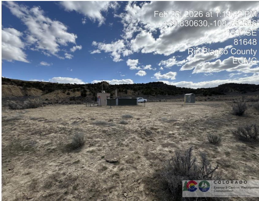
Photo # 2543 NW corner of location
