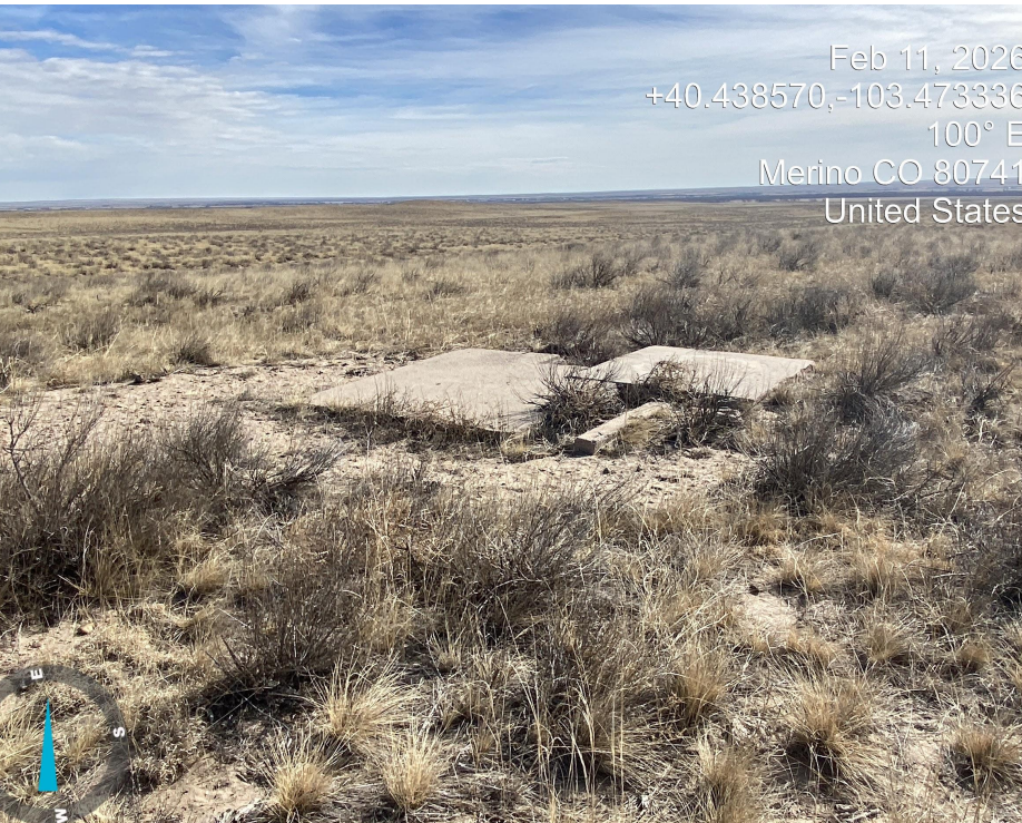
Photo 9. Photo taken from west of the location on the hilltop. The cement pad from that well is still present and needs to be removed. Bare areas present around the pad need to be vegetated with desirable native grass and shrub species.
