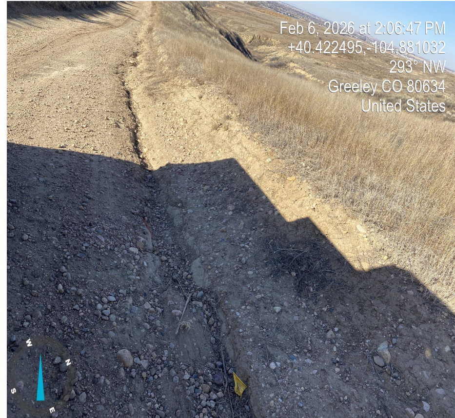
Photo 14. Photo taken from main access road north west past location showing erosion on main road.
