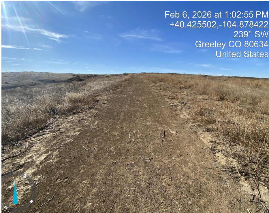
Photo 3. Photo taken from the access road. See the comment in photo 1.
