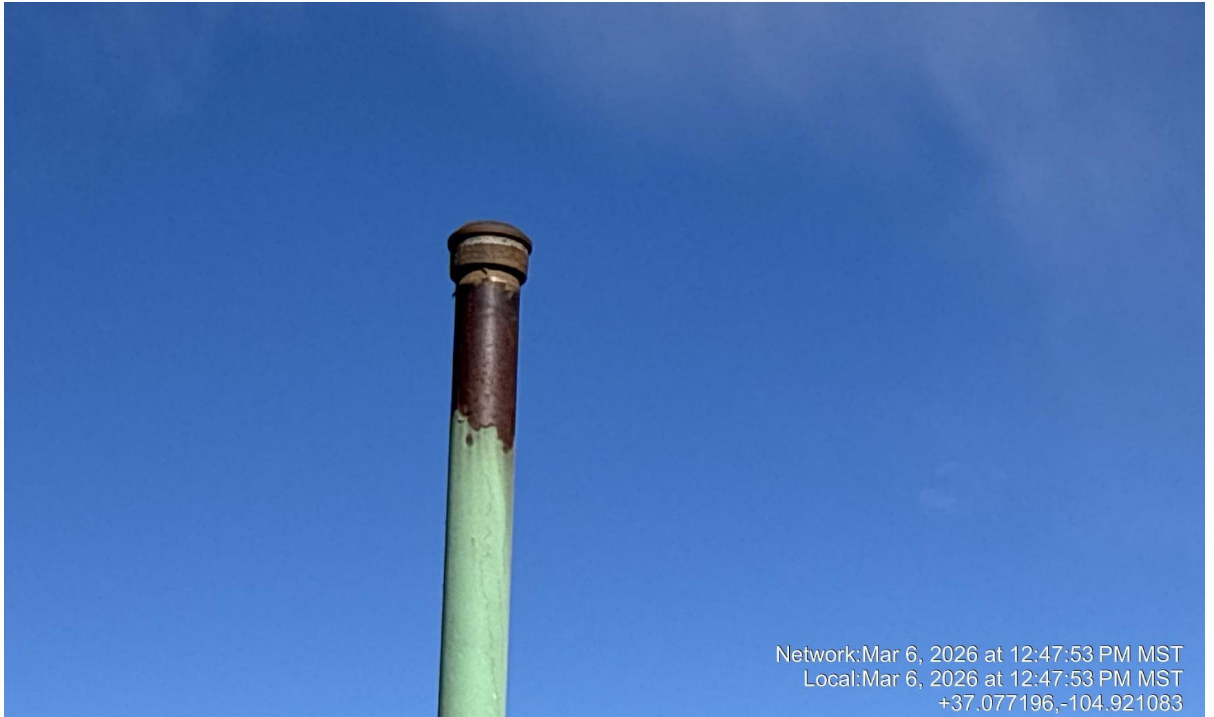
PHOTO 8: Equipment does not properly prevent wildlife entrance or egress (BIRD PROTECTION). Install or repair wildlife protection equipment PER RULE 608.b.(7). CA DATE 3/12/2026.
