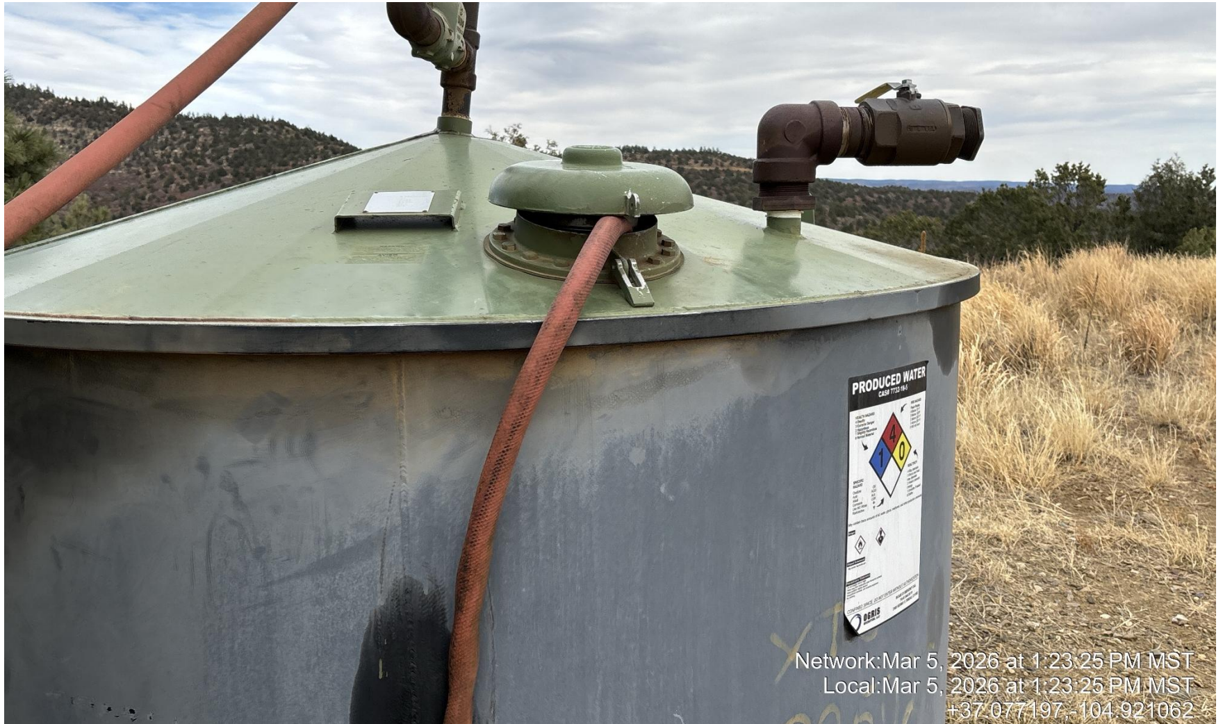
PHOTO 9: Gauge hatch open when not being accessed for gauging or not sealed. Close and seal gauge hatches when not accessing tank per Rule 608. CA DATE 3/7/2026
