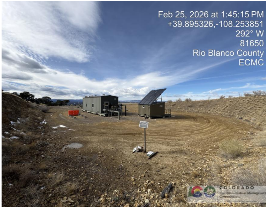
Photo # 2495 SE corner of location
