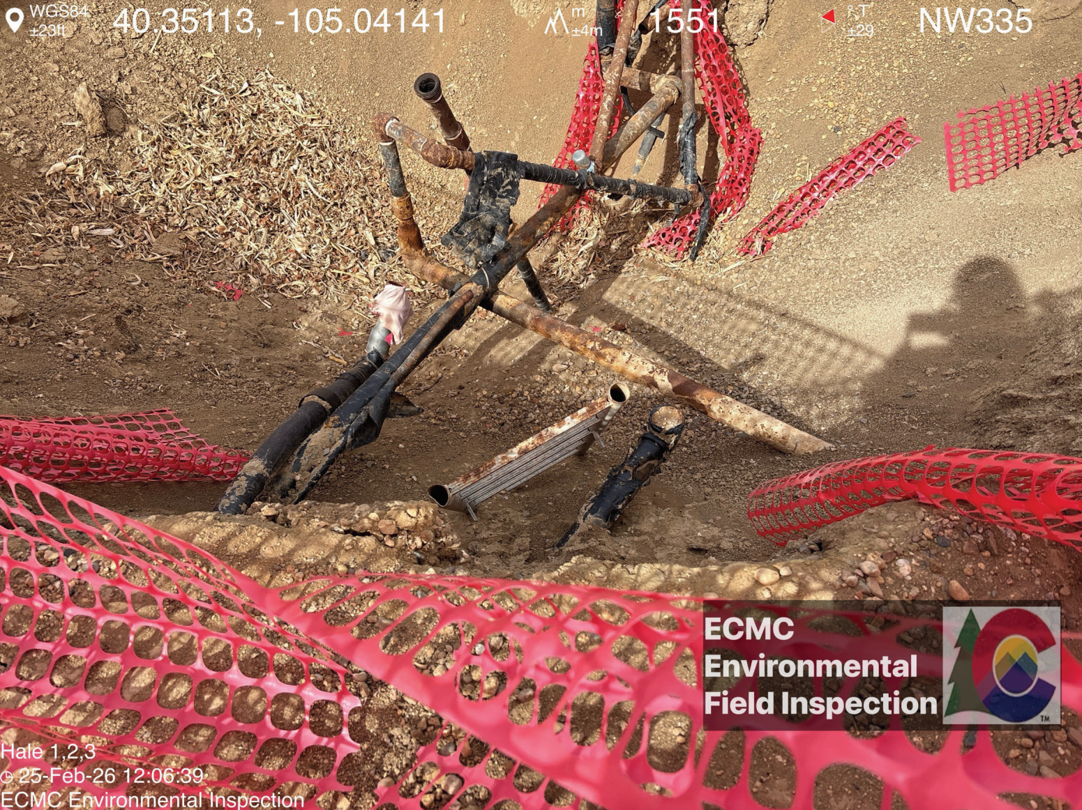
Inadequate fencing, debris (pieces of torn fence), multiple flowlines of unknown status visible within the open excavation at the Hale 3 Separator Spill (Spill ID 488488).
