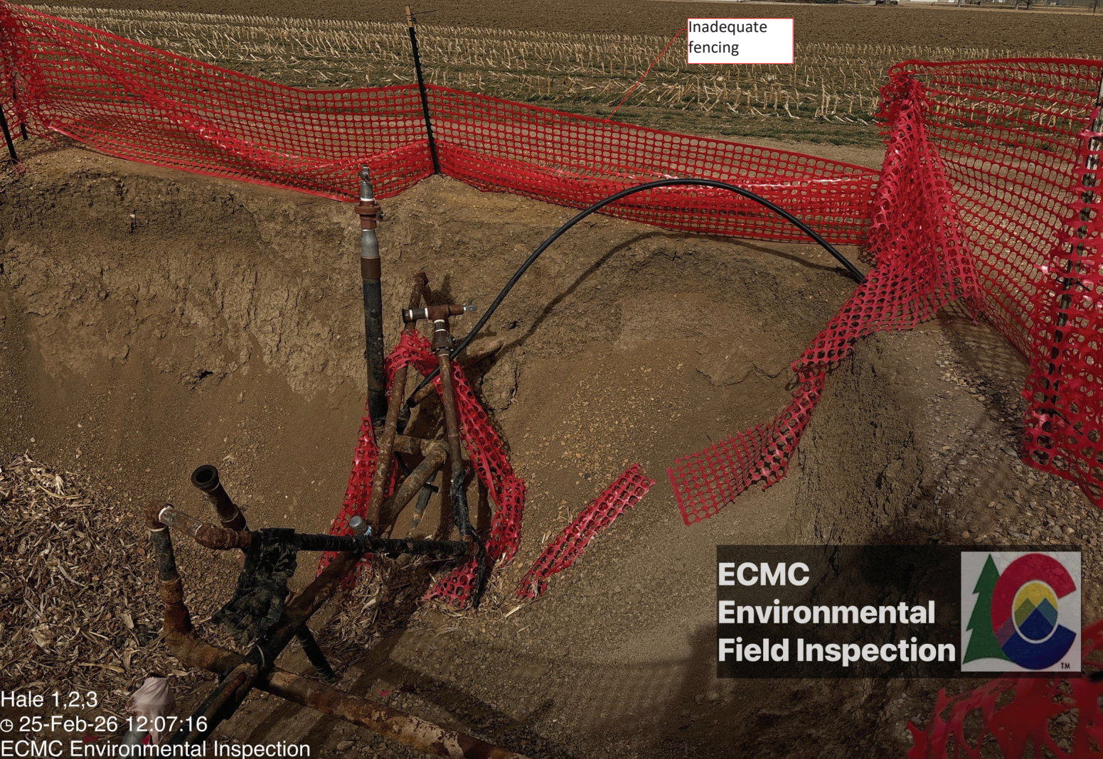
Inadequate fencing, debris (pieces of torn fence), multiple flowlines of unknown status visible within the open excavation at the Hale 3 Separator Spill (Spill ID 488488).
