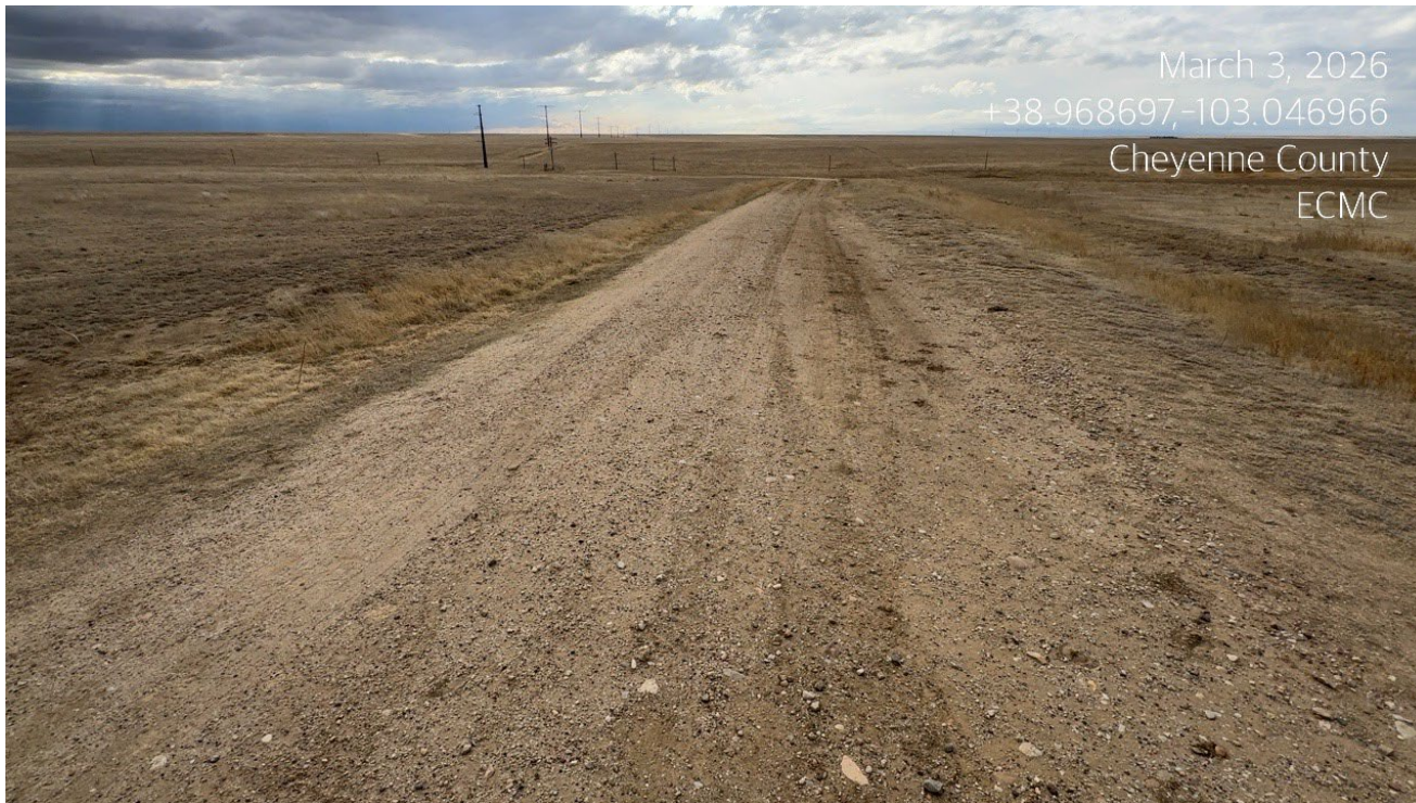
Photo 1. Facing west along the access road. Gravel remains along the road.
