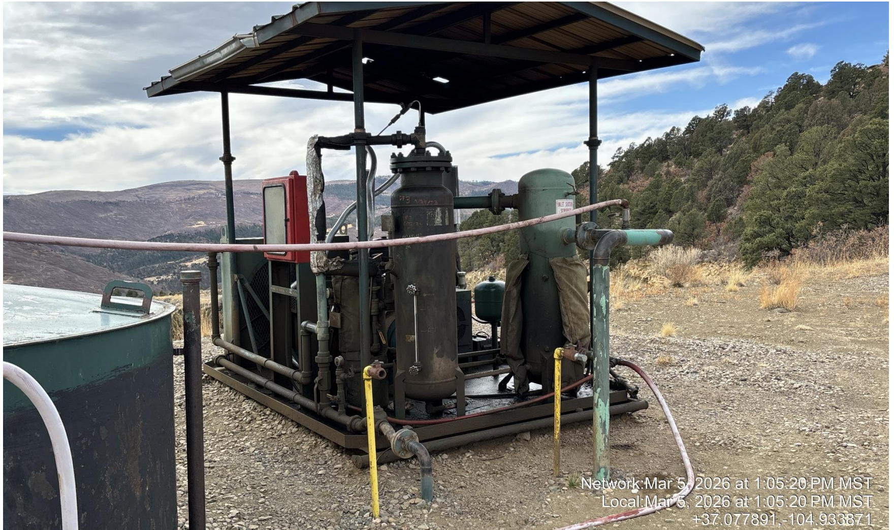
PHOTO 5: Vacuum pump observed on well without ECMC approval. Provide ECMC with documentation showing approval of use of vacuum pump.
