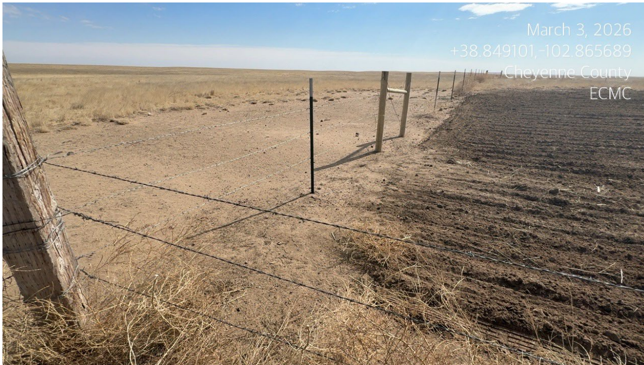
Photo 3. There is an area outside of the fence that was not reclaimed.
