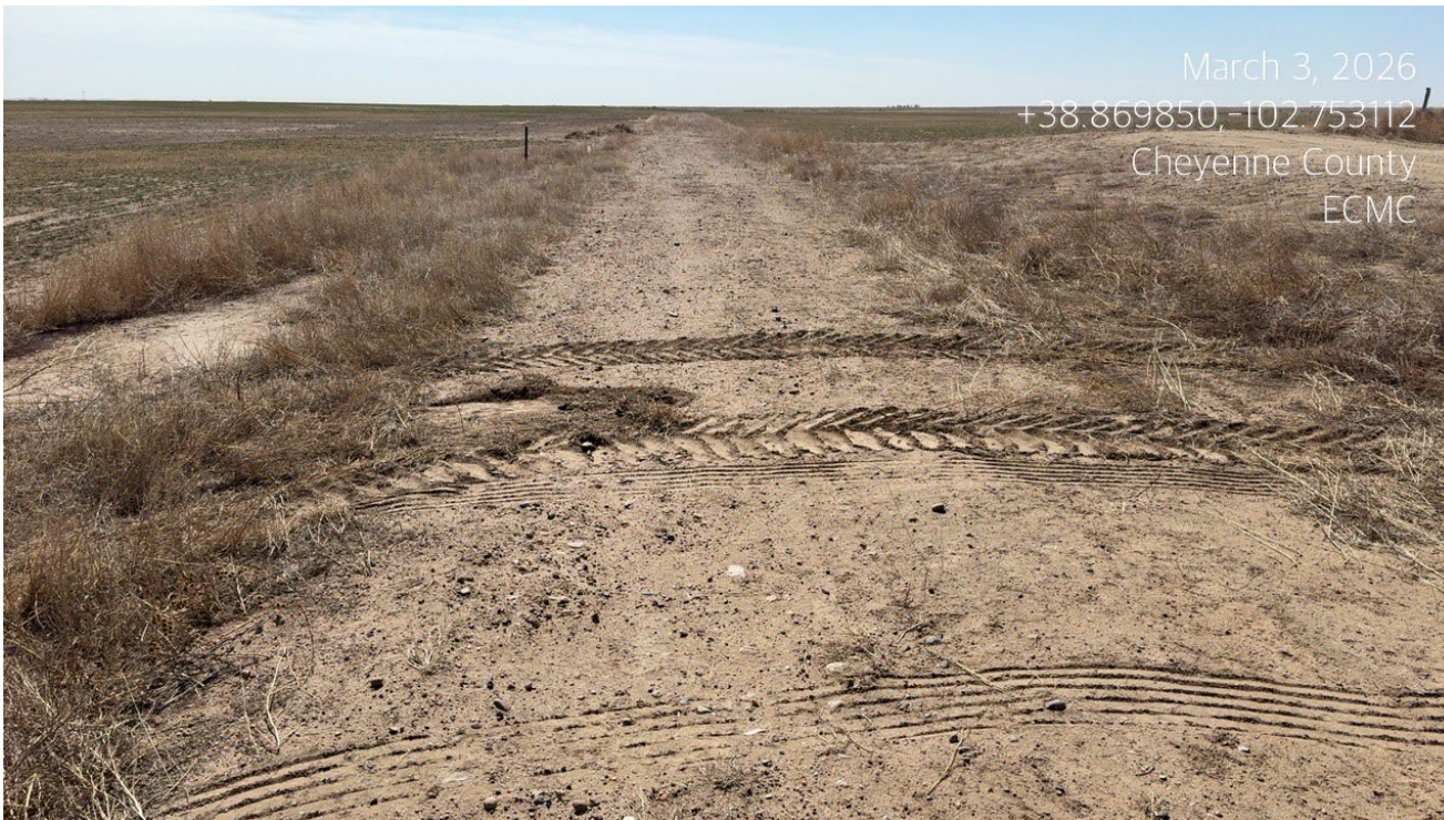
Photo 1. Facing south toward the access road which has not been reclaimed. The gravel road base needs to be removed and soils need to be decompacted by cross ripping to 18 inches.
