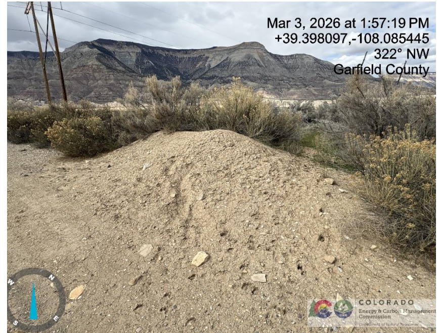
Photo # 5191 Soil stockpile lacks BMP's
