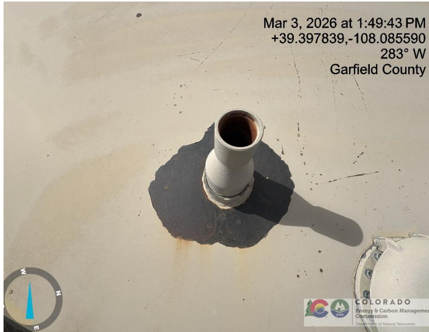
Photo # 5170 Open ended piping on unused production tank /wildlife hazard/available for entry by wildlife
