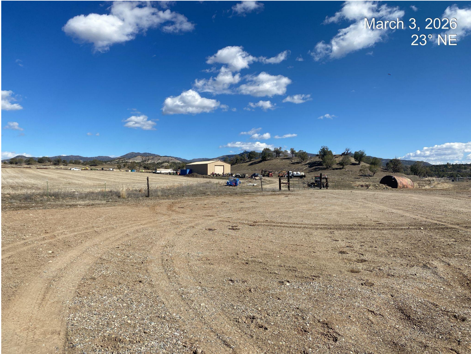
Photo 3. Surface owner equipment has been removed from the working pad surface.
