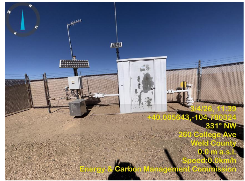
Photo 4 Gas Meter Run, card indicates current calibration.
