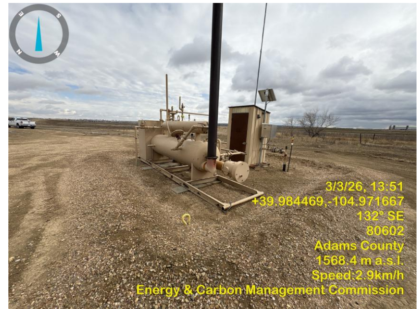
Photo 8 Separator, Gas Meter Run.
