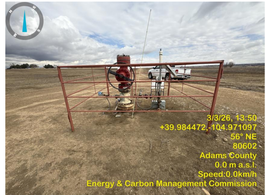
Photo 4 Wellsite, Master valve appears to have a chain & lock.
